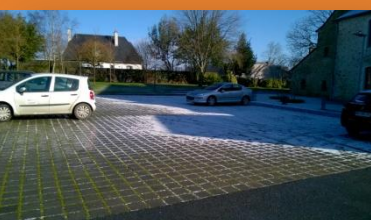
Parking perméable - Loiron
